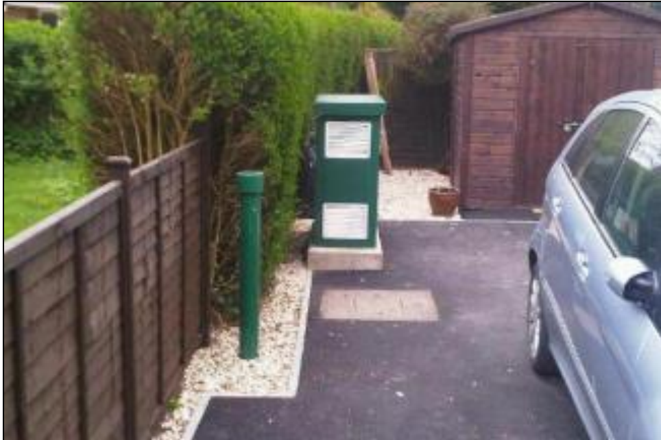
Existing example of low level vent stack pumping stations
