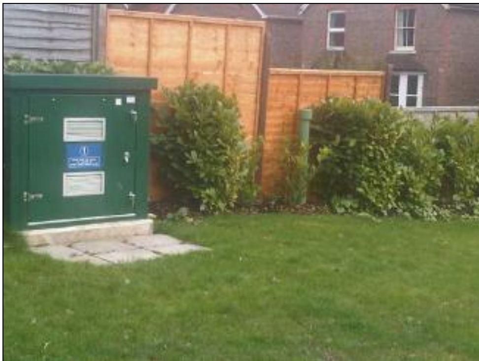
Existing example of low level vent stack pumping stations
